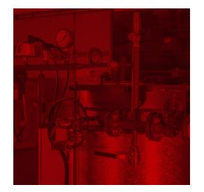
The horizontal GMT and vertical GMT/V steam generators are once-through coil boilers. The exchange of heat between water, steam and combustion products, the relative turbulent regimes, the fluid velocities kept as constant as possible by varying the passage sections, allow to obtain a particularly effective thermal exchange.
