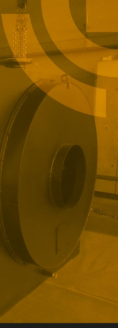
Pressurized steel boiler for hot water production. It can be equipped with a normal market burner and is suitable for liquid or gaseous fuels. Two-position adjustment or, on request, modulating.
